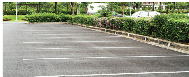
Paved Grounds and Parking Lots
